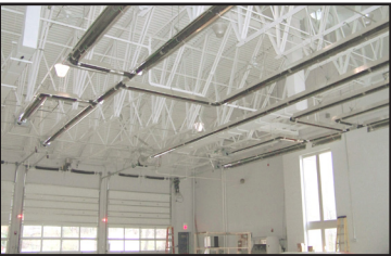
Fire Station Apparatus Bays
